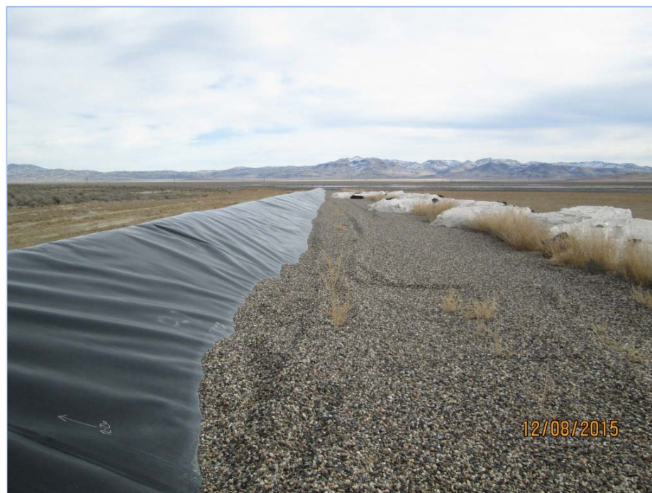
Photograph 0013: Northwest corner of Cell 2 (looking east).
