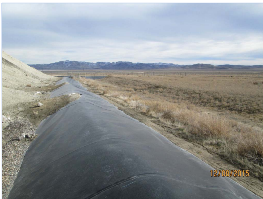
Photograph 0044: Downgradient edge of Cell 1. Stormwater diversion channel is on the right.
