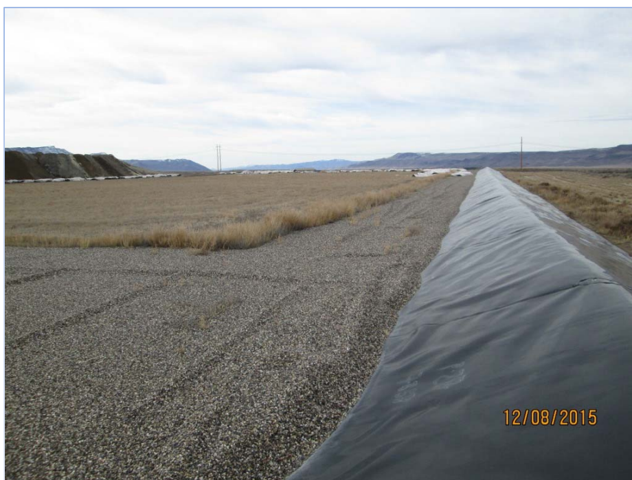
Photograph 0020: Northeast corner of Cell 2 (looking west).
