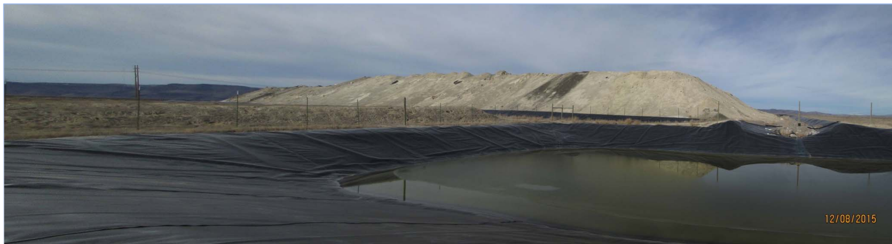
Panoramic Photographs 0067-0068: Typical south side of Cell 1. Collection Pond in foreground.
