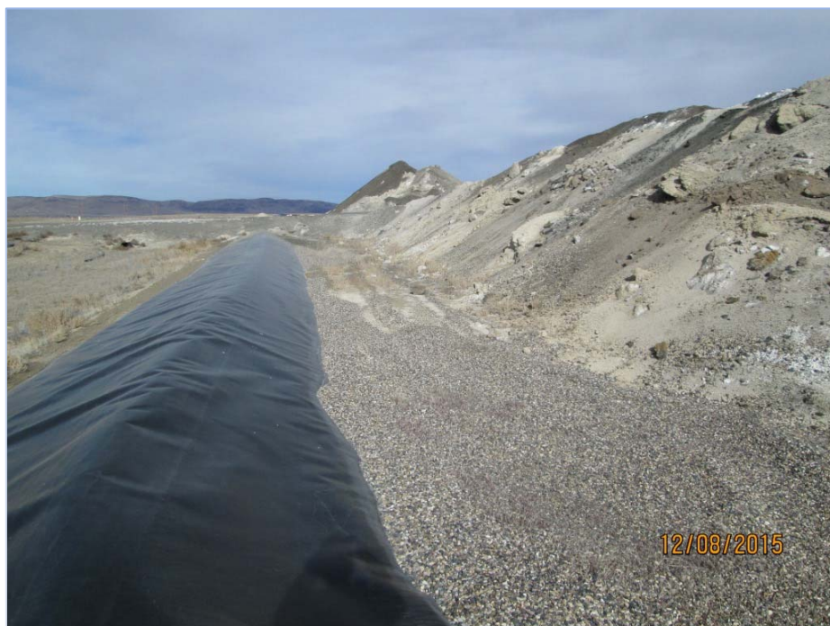
Photograph 0047: Southwest corner of Cell 1 (looking north to access ramp).
