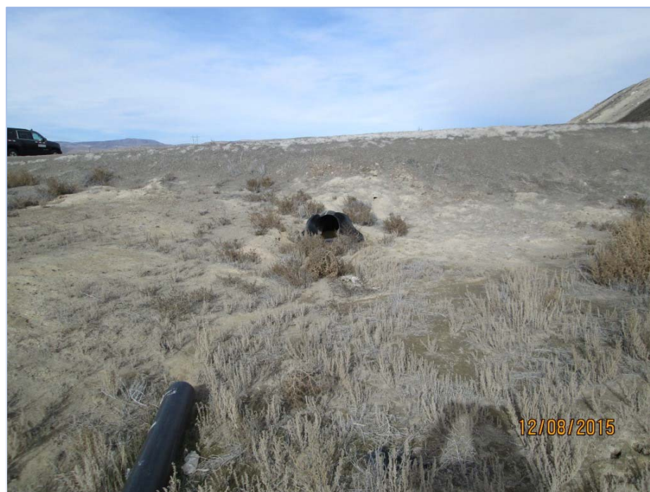
Photograph 0050: Drainage culvert beneath access ramp to Cell 1 (upstream end).
