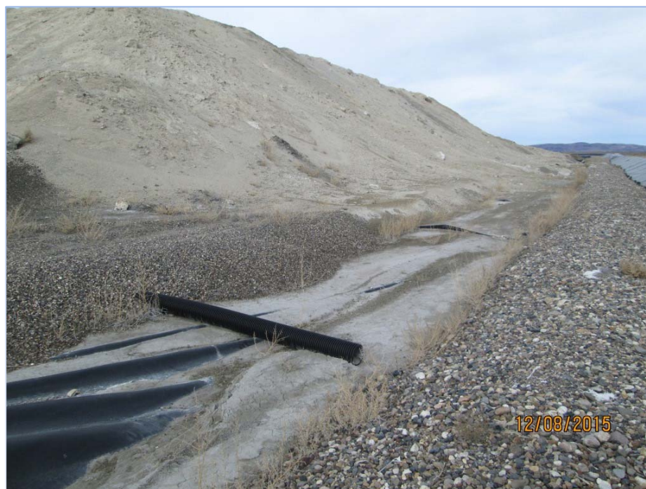
Photograph 0037: Southeast corner of Cell 1 (looking north).
