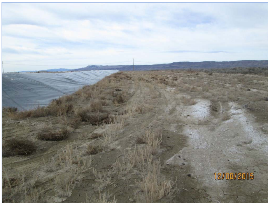
Photograph 0022: Stormwater diversion swale at north side of Cell 2 (looking west).
