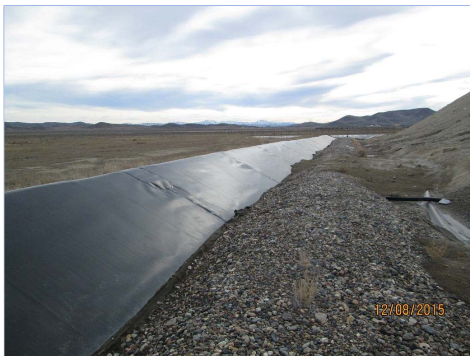
Photograph 0032: Cell 1 collection channel on east side (looking south).
