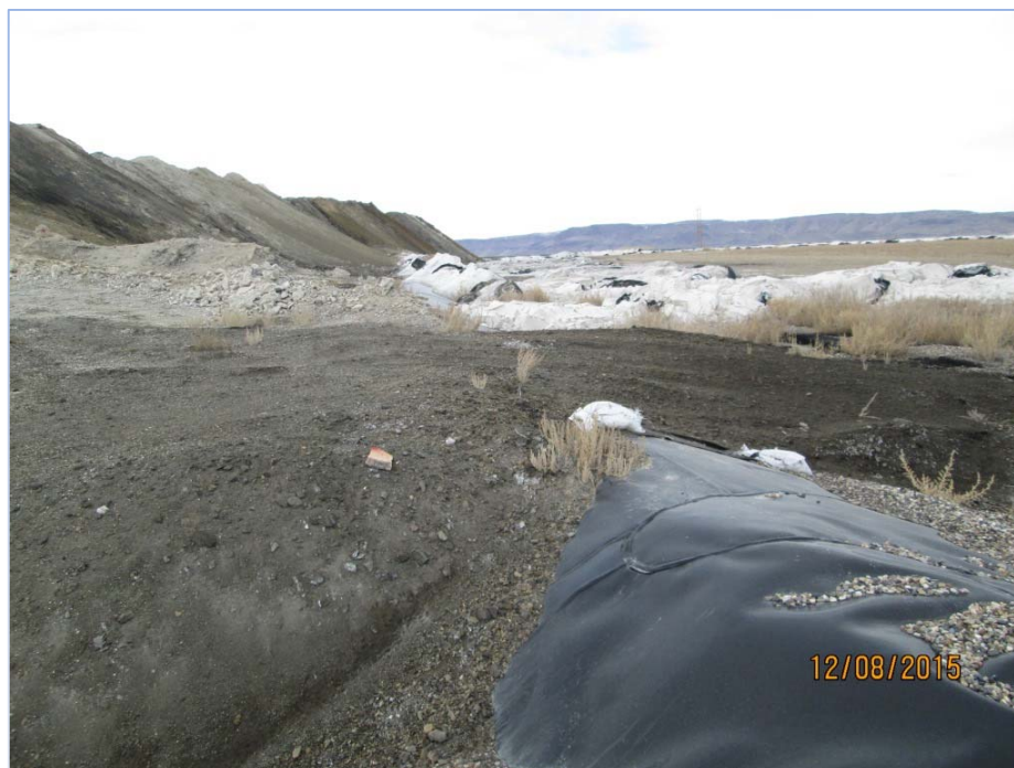
Photograph 0024: Southeast corner of Cell 2 at Cell 1-2 berm (looking west).
