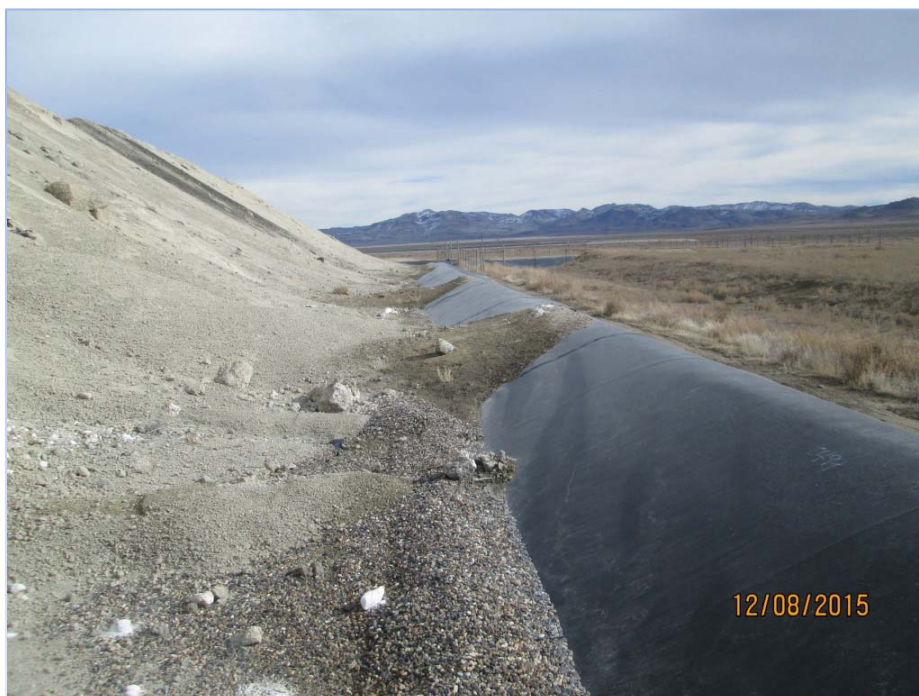
Photograph 0043: South side of Cell 1.
