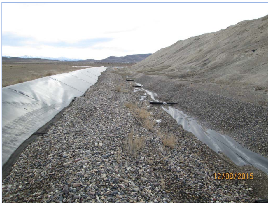
Photograph 0030: Cell 1 collection channel on east side (looking south).
