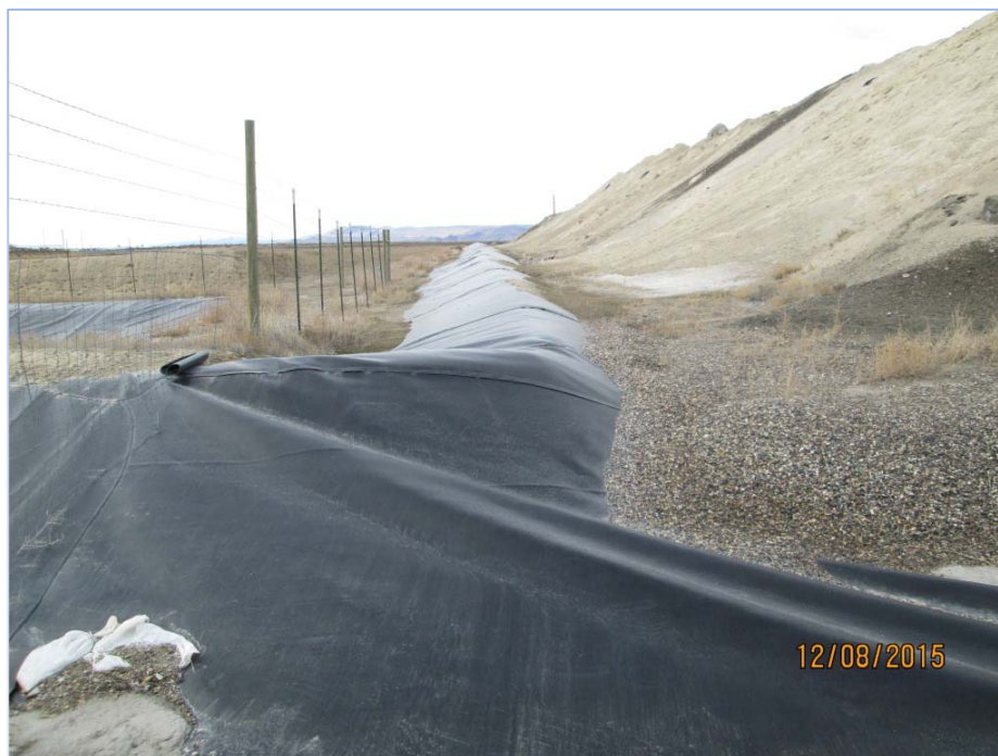
Photograph 0035: South side of Cell 1 at outlet to pond (looking west).
