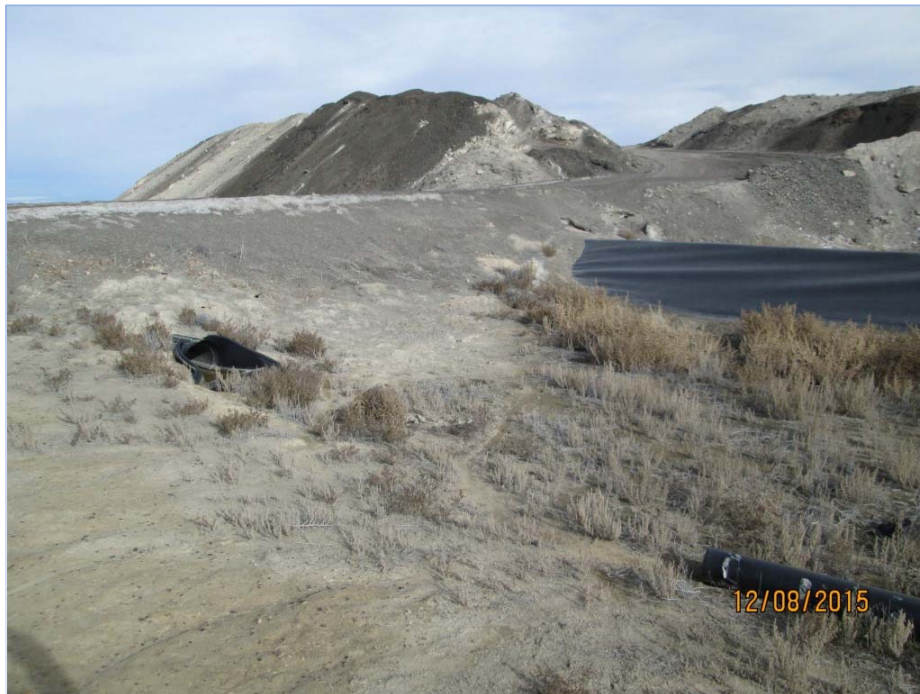
Photograph 0051: Drainage culvert beneath access ramp to Cell 1 (downstream end).
