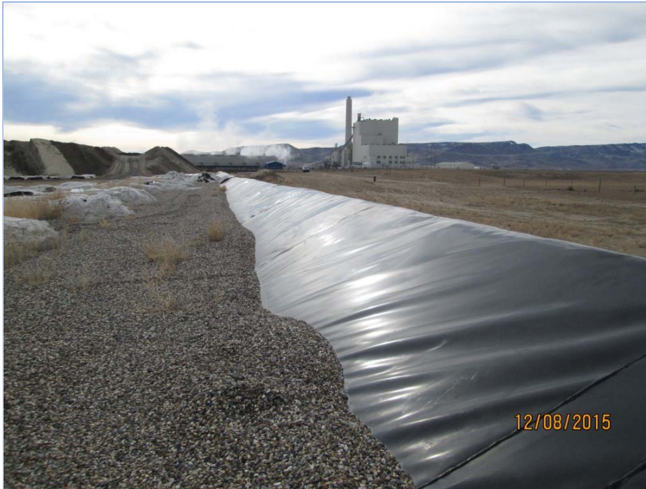
Photograph 0016: Northwest corner of Cell 2 (looking east).
