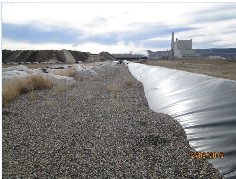
Photograph 0012: West side of Cell 2 near northwest corner (looking south).
