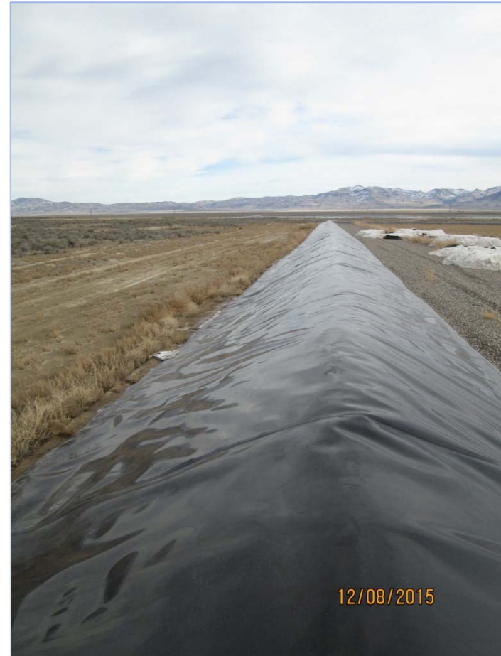
Photograph 0017: North perimeter berm along edge of Cell 2.
