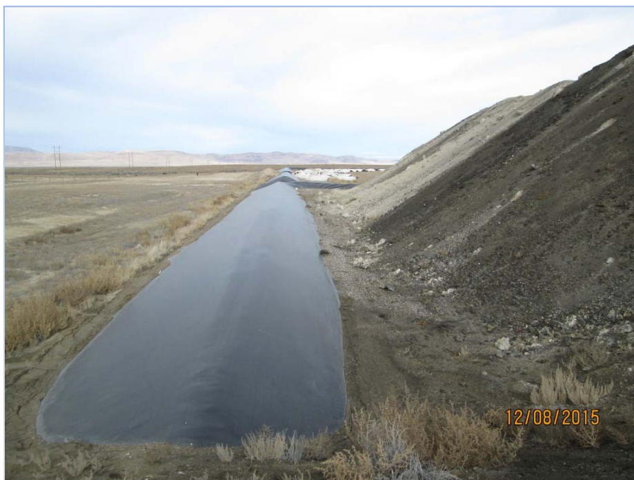
Photograph 0004: West side of Cell 1 north of access ramp (looking north).
